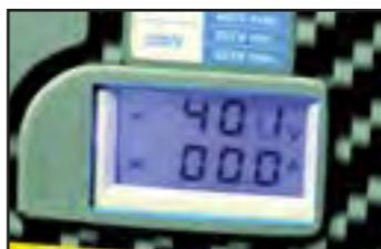
Volts and amps meter control display.
