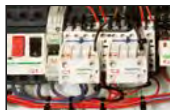
Overload magneto-thermal protection switch.
